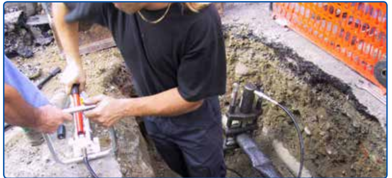
• Pumping operation for pipe compressing
