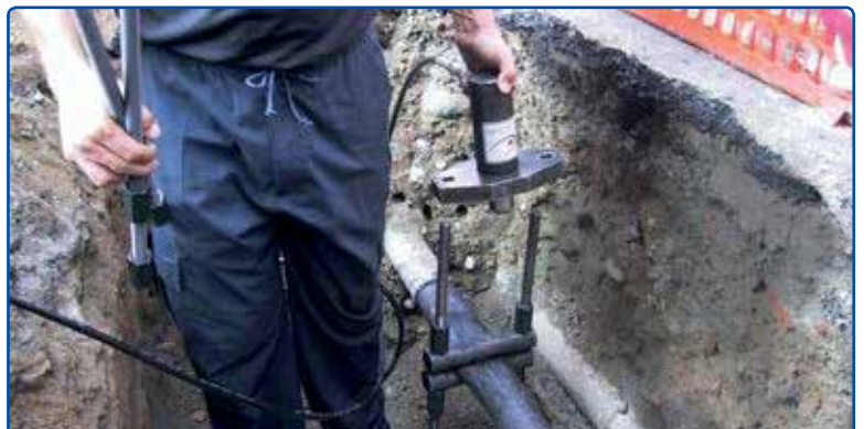
• The cylinder/cross bar group can be detached from the clamp to leave it in compressed mode, the compression operation can be repeated in another point of the pipe with another clamp.
