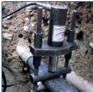
• Pumping operation for pipe compressing
